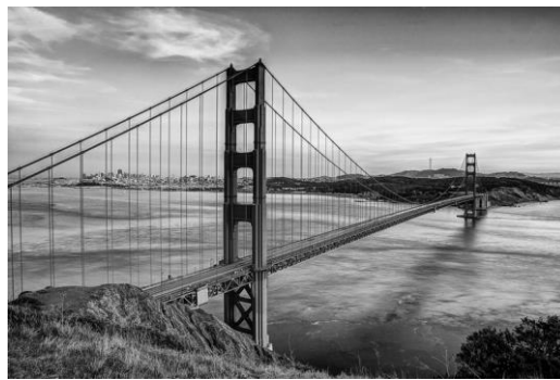
Golden Gate Bridge (金門橋) ～Drawn steel cable (引抜鋼索)～
